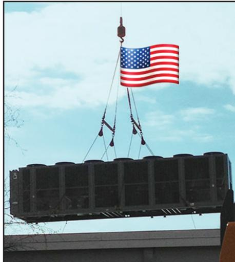
2: Crane lifts the chiller on the roof.
